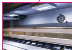
Internal LED Lighting
